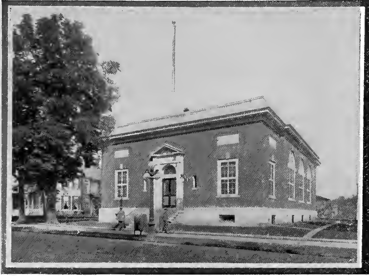
PENN YAN FEDERAL BUILDING.
