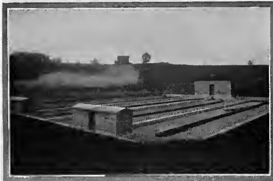
SEWERAGE TREATMENT WORKS.
