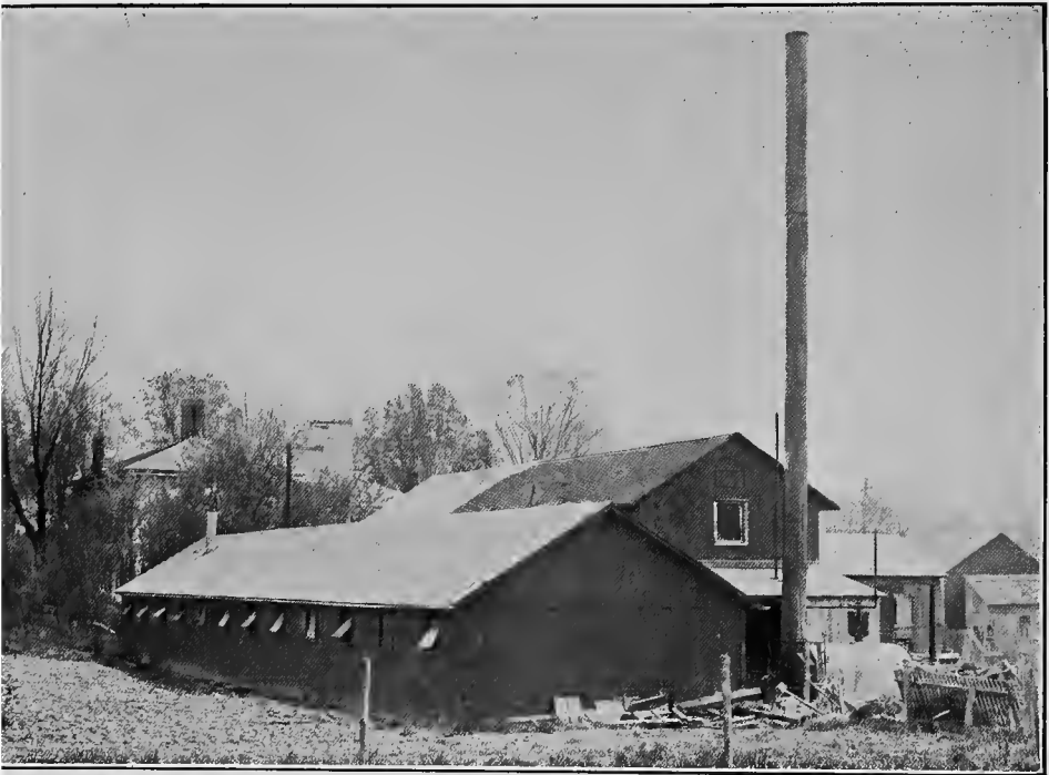
PENN YAN CABLE COMPANY—EXTERIOR VIEW.
