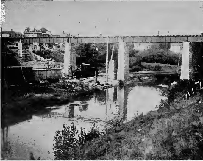
N. C. R. R. BRIDGE CROSSING OUTLET AND N. Y. C. TRACKS.
