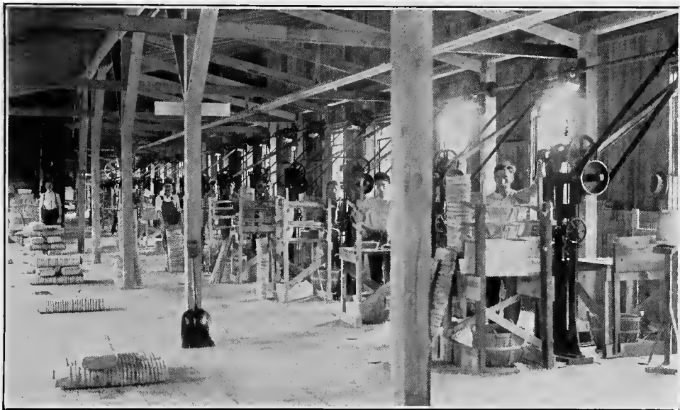
INTERIOR OF BASKET MACHINE ROOM
