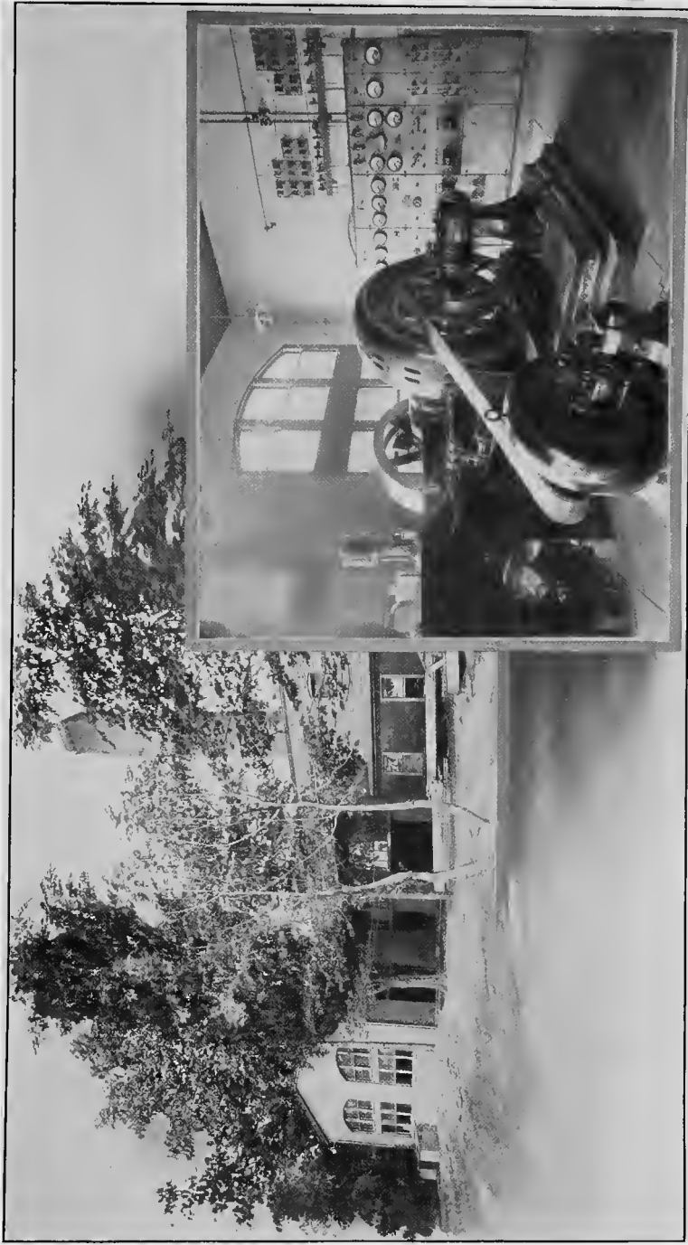
EXTERIOR AND INTERIOR OF MUNICIPAL POWER PLANT. PUBLIC UTILITIES OF PENN YAN. SEE PAGE 56.
